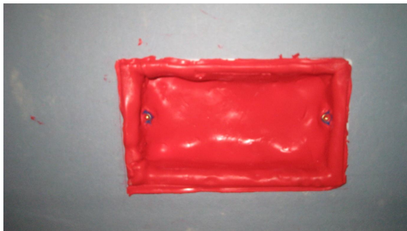
Figure 4 Putty Pad installed inside switch box
