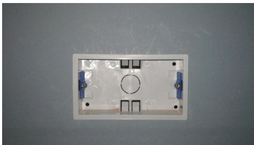
Figure 3 Switch box before installation of Putty Pad
